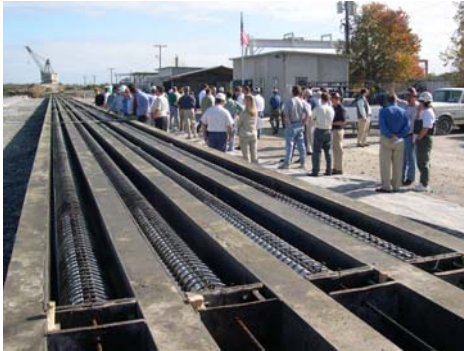
Casting Beds with Spiral Strands in place
