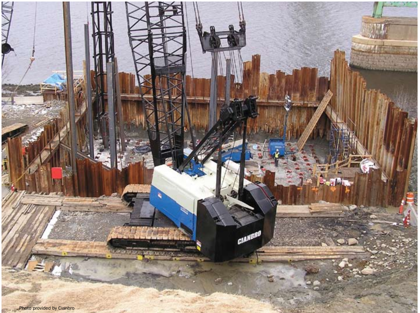
Photo provided by Cianbro
