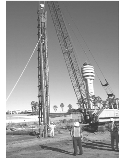
Crane and pile driving rig
