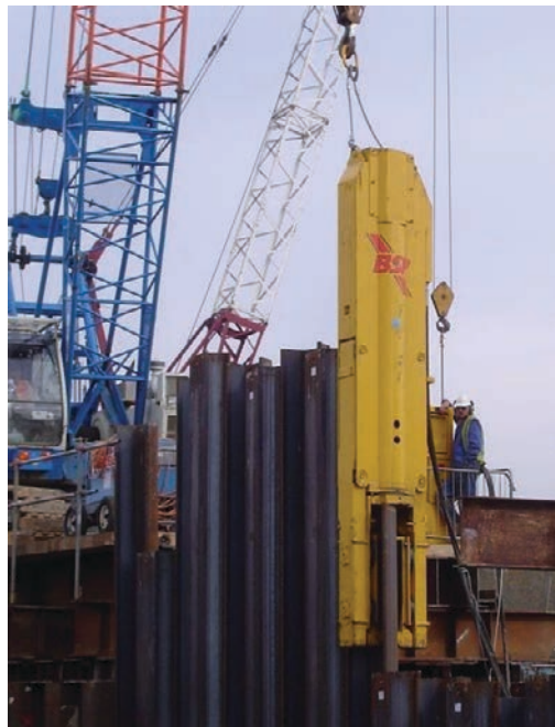
Crane suspended hammer
